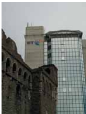
Figures 41/42 The BT building
