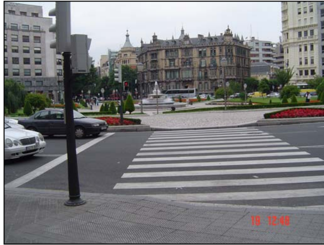
Figure 2: Signalised Gyratory with pedestrianised central island, Central Bilbao
