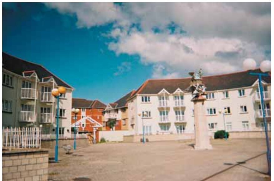
Figure 32 Lighting at the marina seafront
