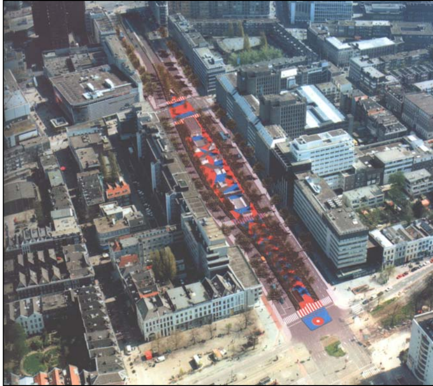
Figure 4: Example of Boulevard, Rotterdam
